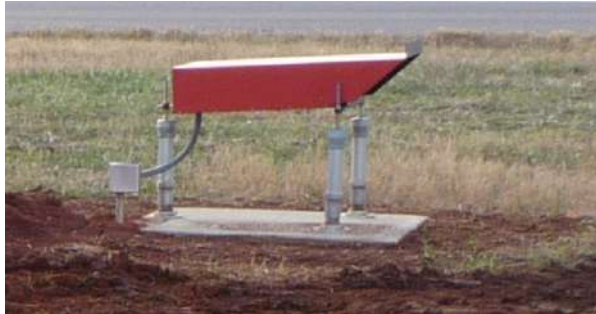
Example Of An Installed LHA
