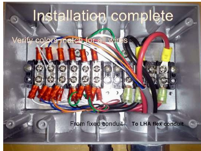
Figure 11: Junction box with final connections (note: tilt switch connections not shown)
